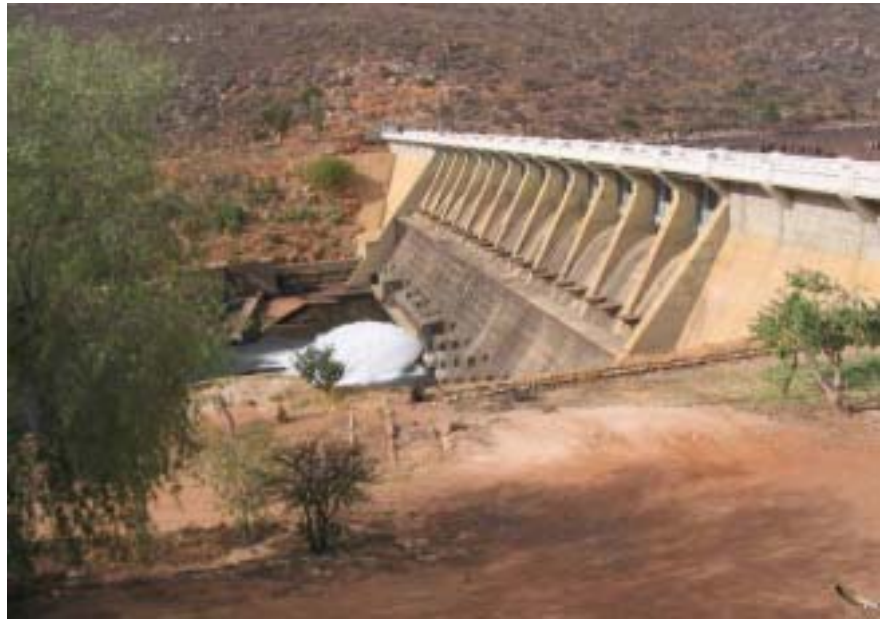
The existing Clanwilliam Dam wall
