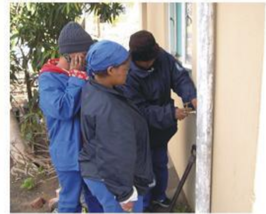
The ladies of the Clanwilliam leak repair team hard at work replacing a leaking tap.
