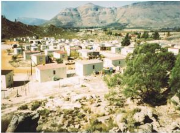
The high density housing suburb of Op-die-Berg Koue Bokkeveld. A large number of leaks were found here.
