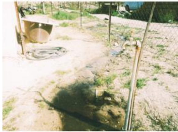
In the most severe instance a leak accounted for almost 350kl water consumed per month
