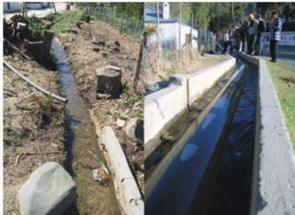
In Wupperthal water loss is experienced due to many cracks and seepage along the canal. The micro-project uses a cost effective, lay-flat pipe to conserve water while creating greater awareness.
