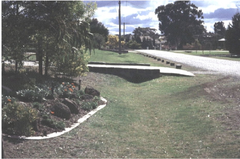
FIGURE 8: GRASS SWALES IN PLACE OF THE TRADITION KERB AND CHANNEL SYSTEM FOR MANAGEMENT OF ROAD RUNOFF CAN PROMOTE BOTH WATER QUALITY IMPROVEMENT AND FLOW ATTENUATION.
